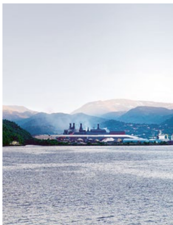
Silicon-metal production site in Holla, Norway
